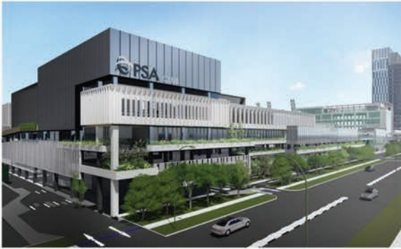
PSA CORPORATE HEADQUARTERS Pasir Panjang Avenue 7, Singapore
